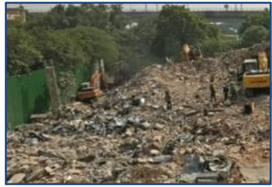
November 2018 Existing building demolished; construction started
