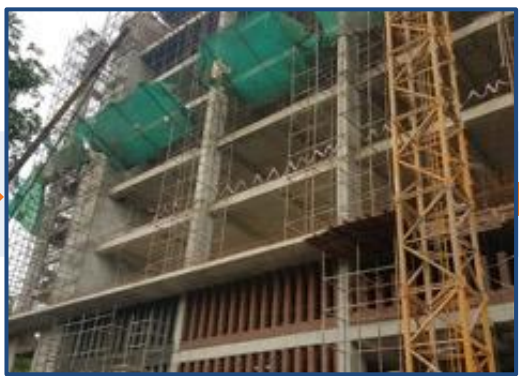
June 2019 Structure completed upto L6
