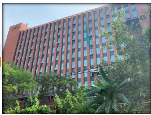
June 2020 Glass Façade Completed
