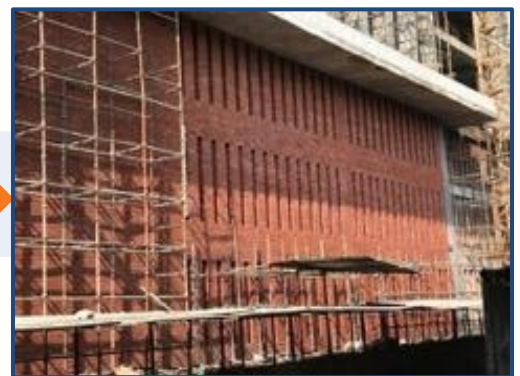
September 2019 Structure completed
